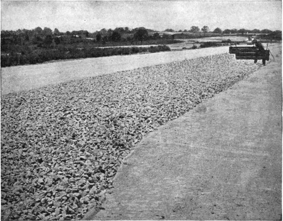
Figure 75. Macadam base course under construction.
